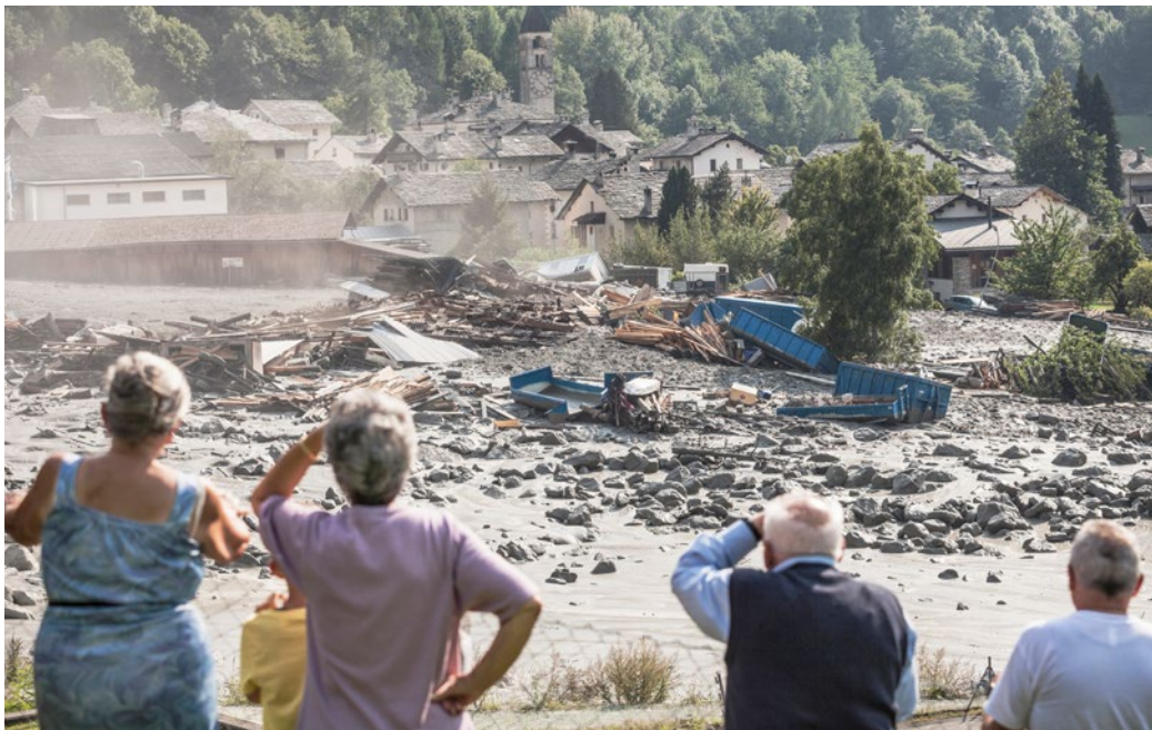
Bondo residents survey the destruction caused by the avalanche of mud, debris and scree on 23 August.
